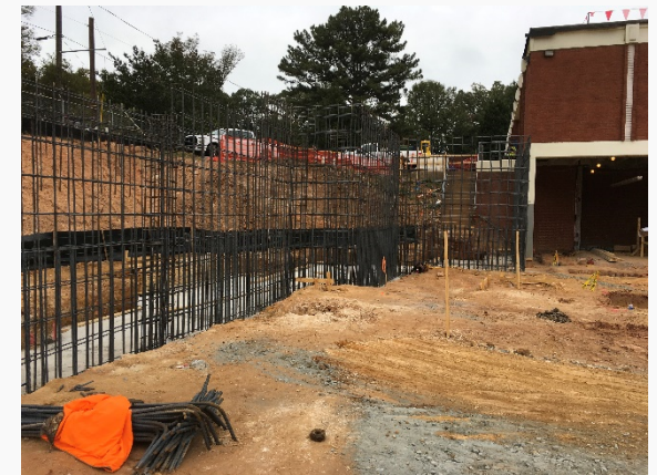
Installation of wall rebar
