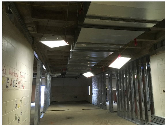
Interior MEP Rough and framing at renovation
