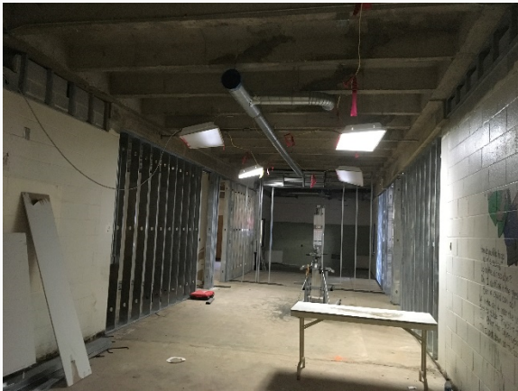
Interior MEP Rough and framing at renovation
