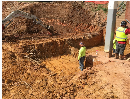
Survey Layout and Footing Excavation
