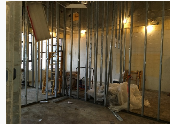
Renovation Framing and MEP Rough
