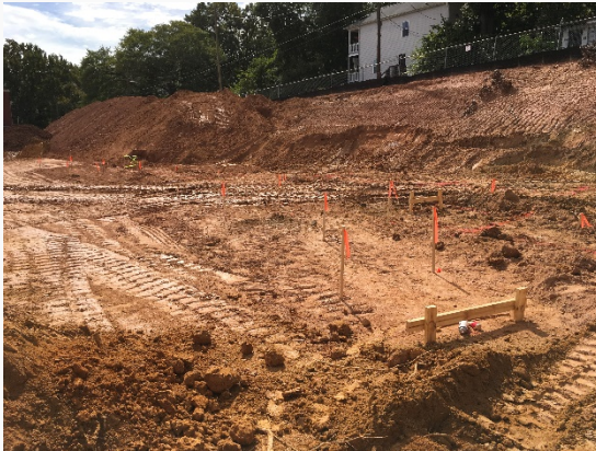
Survey Layout and Footing Excavation
