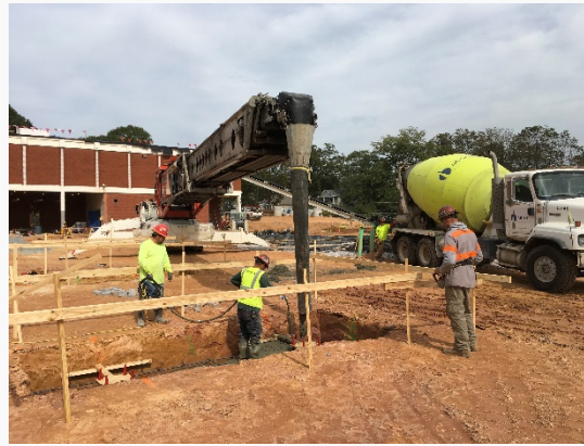
New Building foundations and wall formwork
